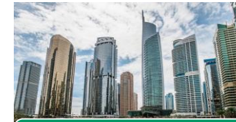
Jumeirah Lake Towers 150k RT
